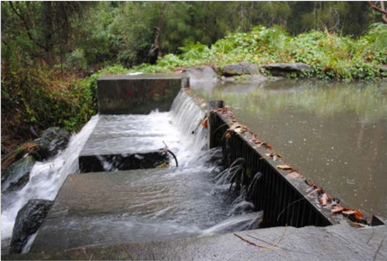
Photo 3: Warringah drain with rudimentary control, capturing organic matter. Photo by Aaron Wright, DPIE–EES
